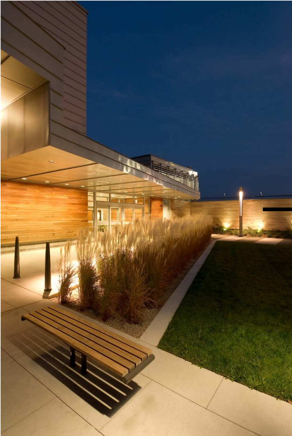
THE WOOD CLADDING CONCEALS THE AIRPORT BLAST WALL AND BARBED WIRE
