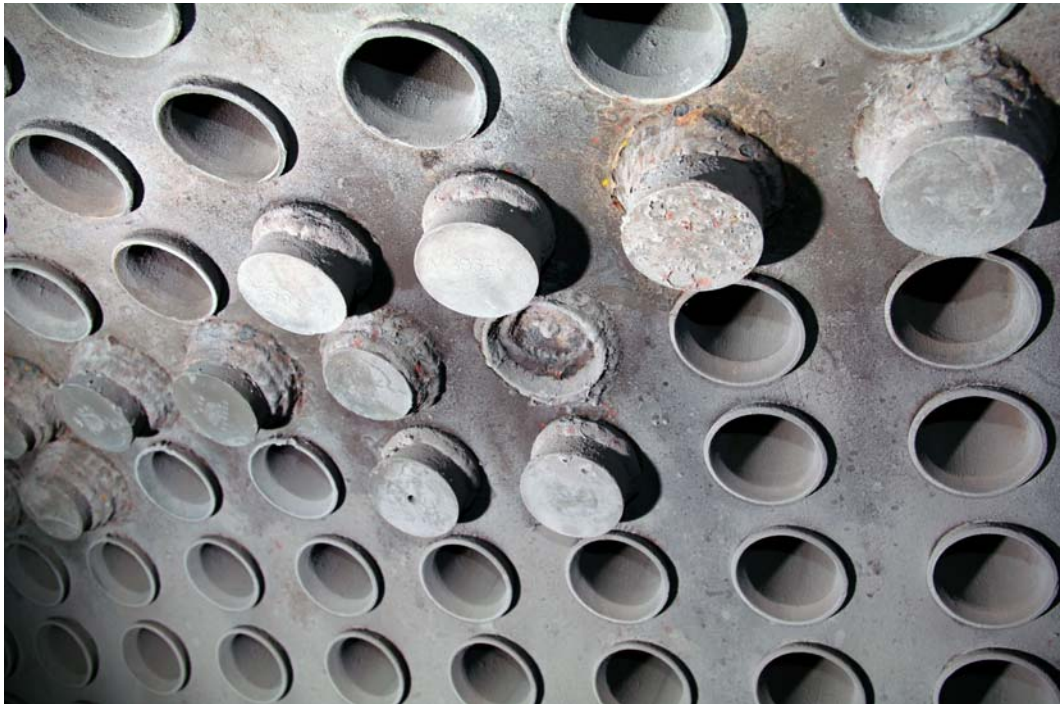
FIGURE 28. Mud drum plugged tubes.
