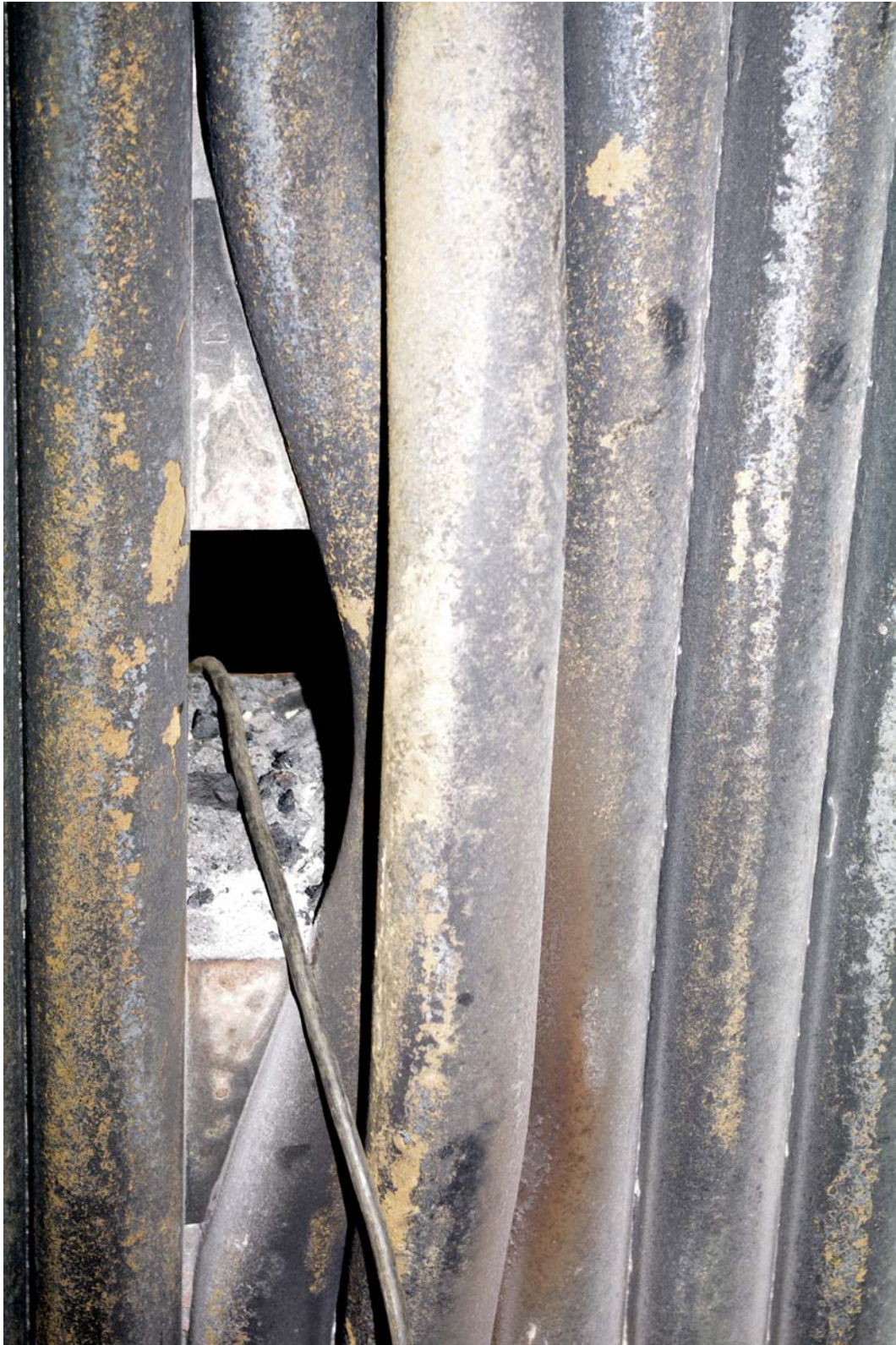
FIGURE 11. Inspection port tubing appears to be in good condition.
