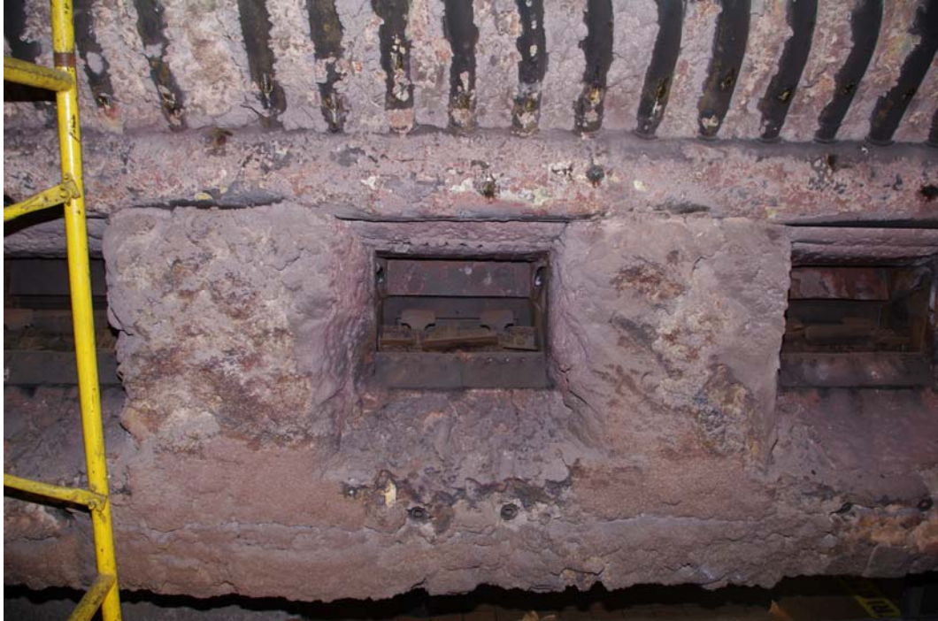
FIGURE 7. Front wall of the furnace showing spreader paddles.
