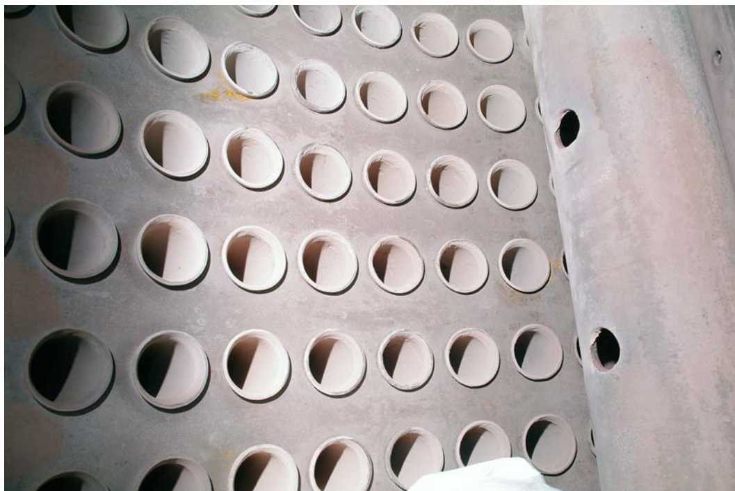
FIGURE 21. Steam drum tubes.
