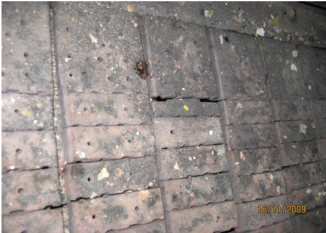
FIGURE 8. Grating evidences link wear producing gaps.
