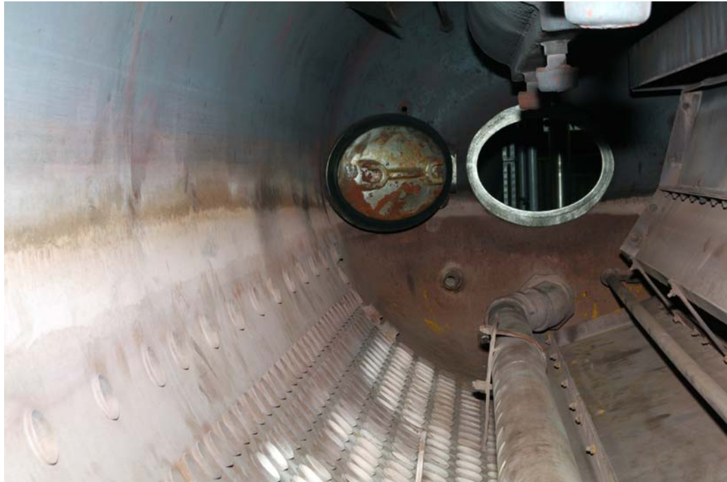
FIGURE 19. Steam drum internals.
