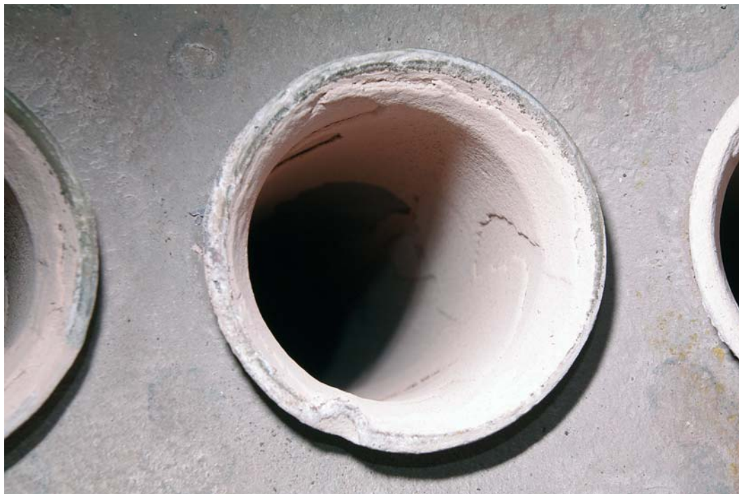
FIGURE 22. Representative tube as seen from the steam drum.
