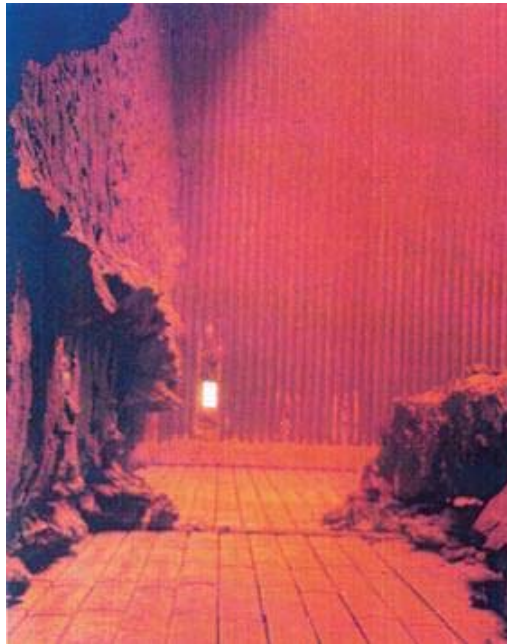
Figure 8-5 Biomass Boiler Slagging After Operating for 4 Days on Urban Tree Trimmings (Source: T.R. Miles)
