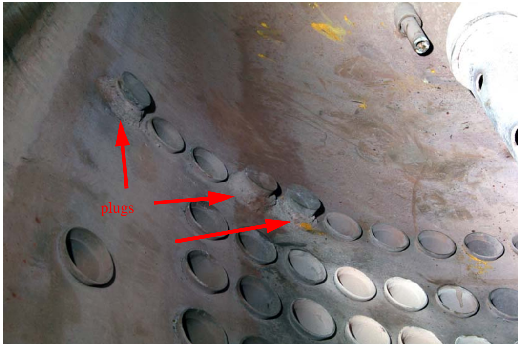
FIGURE 23. Steam plugged tubes.
