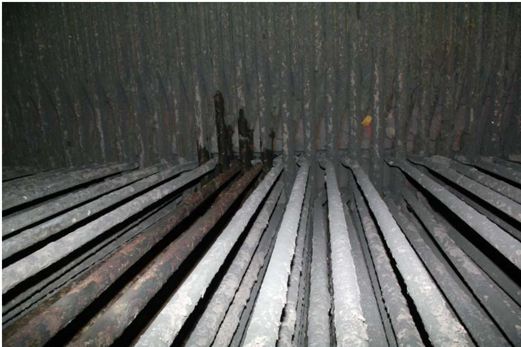
FIGURE 15. Superheater pendant showing loose alignment.
