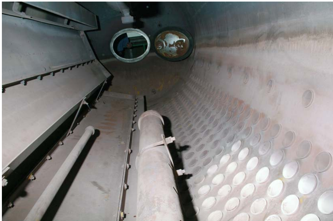
FIGURE 20. Steam drum internals in the opposite direction.
