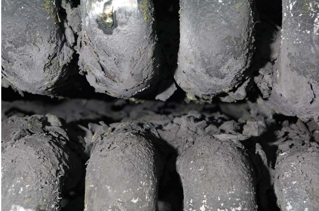
FIGURE 34. Close-up of economizer loops with significant blockage between tubes.
