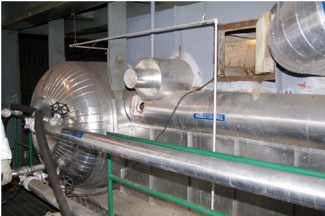
FIGURE 4. Outside view of steam drum and penthouse entrance.
