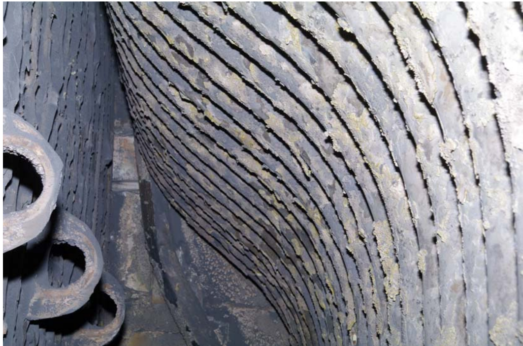
FIGURE 24. Generating bank tubing.
