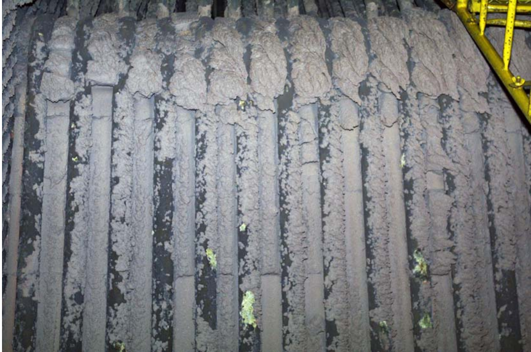
FIGURE 14. Rear wall at nose, note slag build-up.
