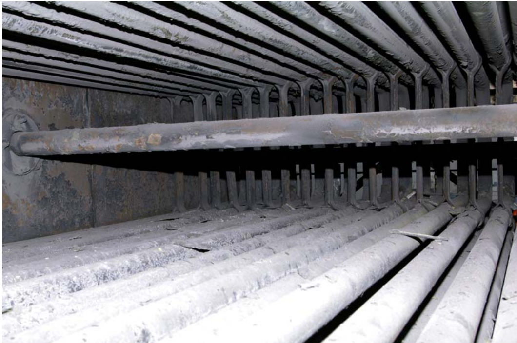
FIGURE 35. View from inside the middle section of the economizer.
