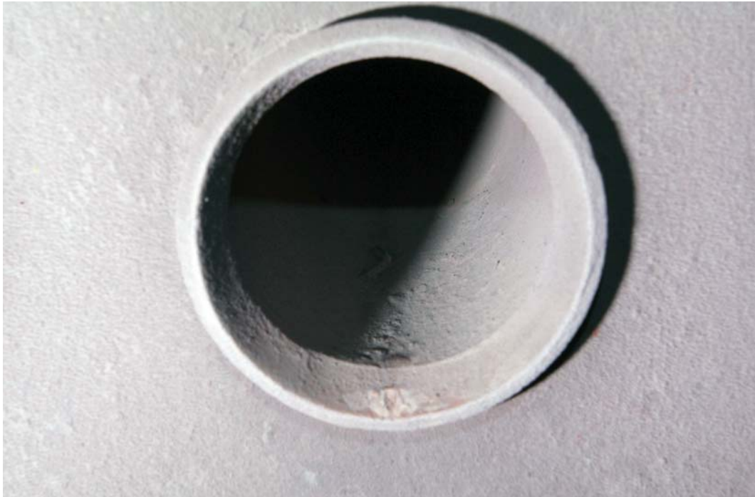
FIGURE 29. Representative tube as seen from the mud drum.
