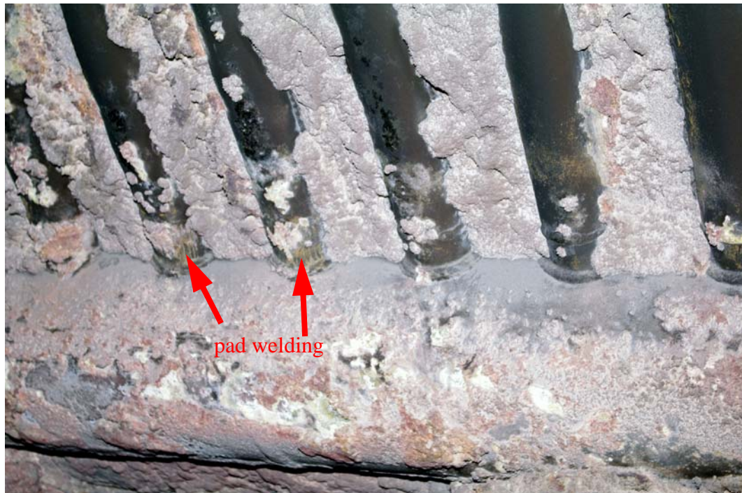
FIGURE 9. Front wall header connection with evidence of pad weld repairs.
