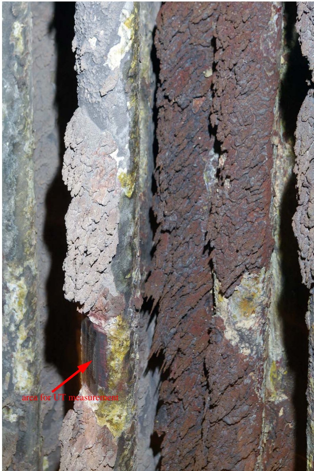
FIGURE 18. Close-up of superheater pendants, note area prepped for UT thickness measurement.
