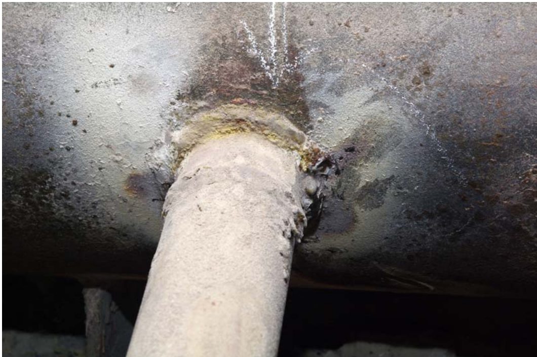
FIGURE 32. Header to tube repair.
