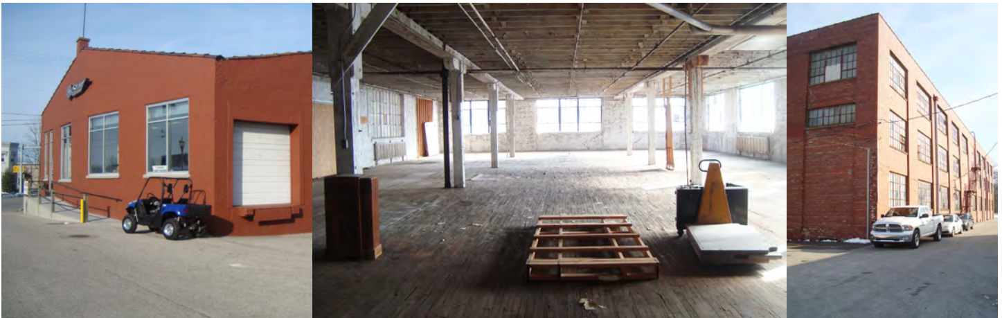
The Hoosier Desk property contains approximately 130,000 square feet of usable space. Its configuration and location suggests a redevelopment plan composed of a mix of retail, restaurant, and arts and cultural spaces on its first floor, with residential units on its upper floors. Ample parking can be provided on-site.
