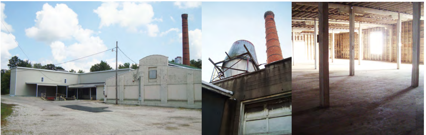
Above: The Veneer Mill is 58,000 square feet on two floors. The conceptual plan suggests this property primarily be redeveloped as a mix of restaurant space and residential units. The upper floor layout appears to be particularly adaptable for apartments.
