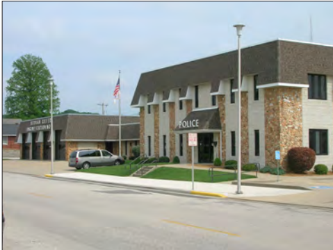
Police and Fire Station Headquarters on 6th Street
