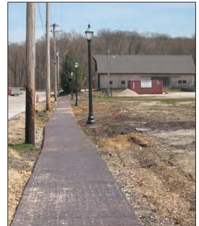
New decorative sidewalk and streetlight project along 4th Street
