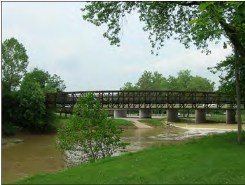
The Riverwalk Bridge over the Patoka River
