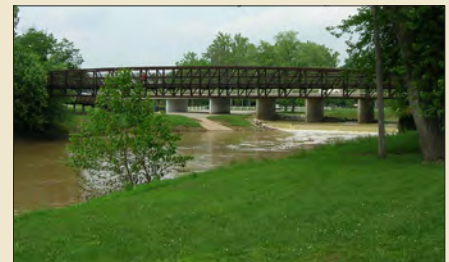
The Patoka River at the 3rd Avenue Bridge
