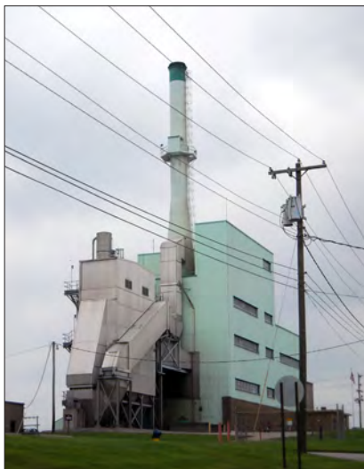
15th Street Electrical Station
