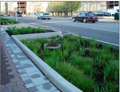
Curbside rain garden collects and filters stormwater runoff
