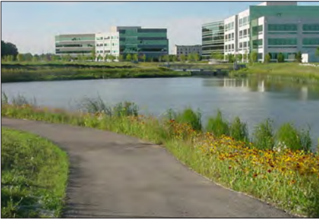
Shared stormwater facility as a site amenity within this office park
