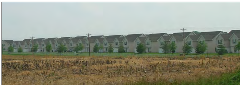
Multi-family housing along U.S. 231 near 47th Street
