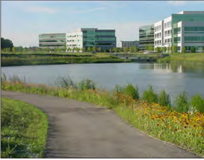
Shared stormwater facility is also a site amenity
