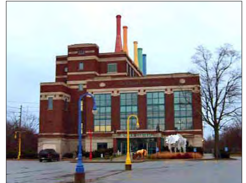
Reuse of a former power plant into a children's museum in Ft. Wayne, IN
