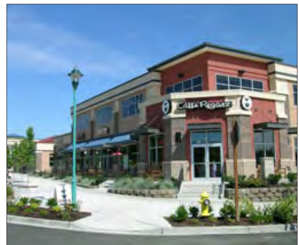
Two photos above illustrate buildings with facade details such as awnings, canopies, roof detail, a variety of materials, cornices and pedestrian scale externally illuminated signage. Landscaping and site furnishings add pedestrian comfort.
