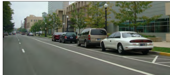
Example of a one-way street with two travel lanes, a bike lane, and on-street parking.
