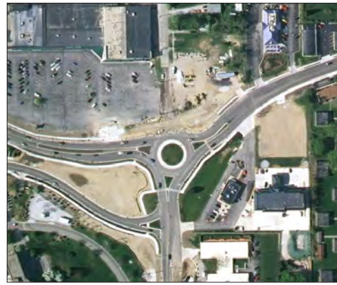
Construction of a roundabout at the intersection of two state highways in Valparaiso, IN
